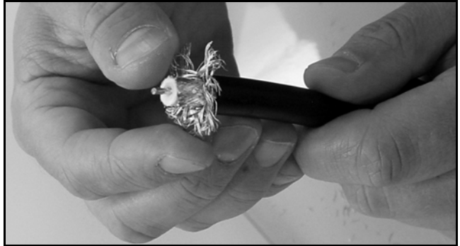
Figure 71: Flaring the Braid
