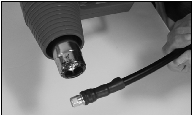
Figure 97: Applying the Heat Shrink Tubing
