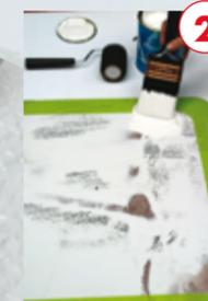
Apply and spread KiwiGrip onto the prepped surface. KiwiGrip can even be applied on top of other non-skid surfaces.
